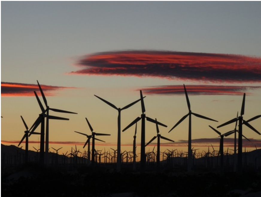
Palm Springs wind farm. (Photo: Liisa Atva)
